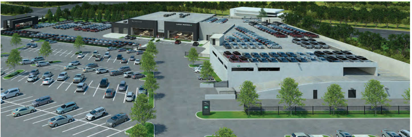
Future home of Jaguar Land Rover Portland now under construction at Washington Square
